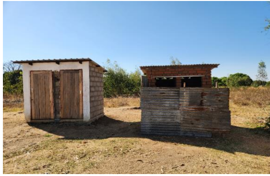
Figure 9: A MK4.5 Million Pit latrine (Left) under Commercial Contracting vs a MK87,000 Pit latrine built by the community contracting (right)
