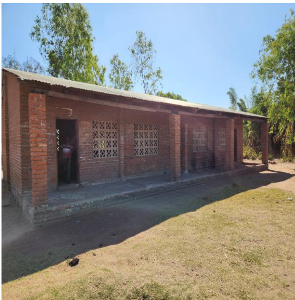
Figure 7 : A MK46 Million Classroom block built over a period of 3 years.
