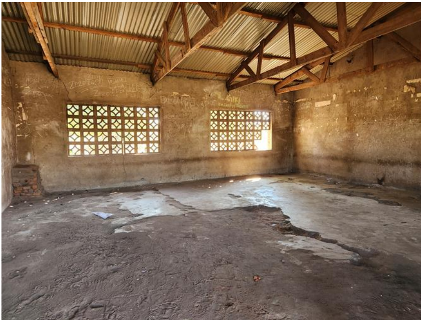
Figure 8: Picture showing the interior of a MK46,000,000 school block constructed under commercial contracting
